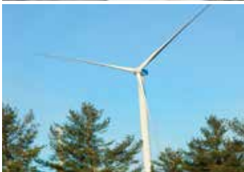
Renewables in Nova Scotia: Sissiboo Hydro (top) and South Canoe wind farm (bottom).
