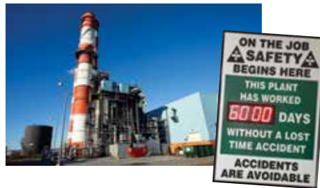
Emera Energy's Bayside plant.
