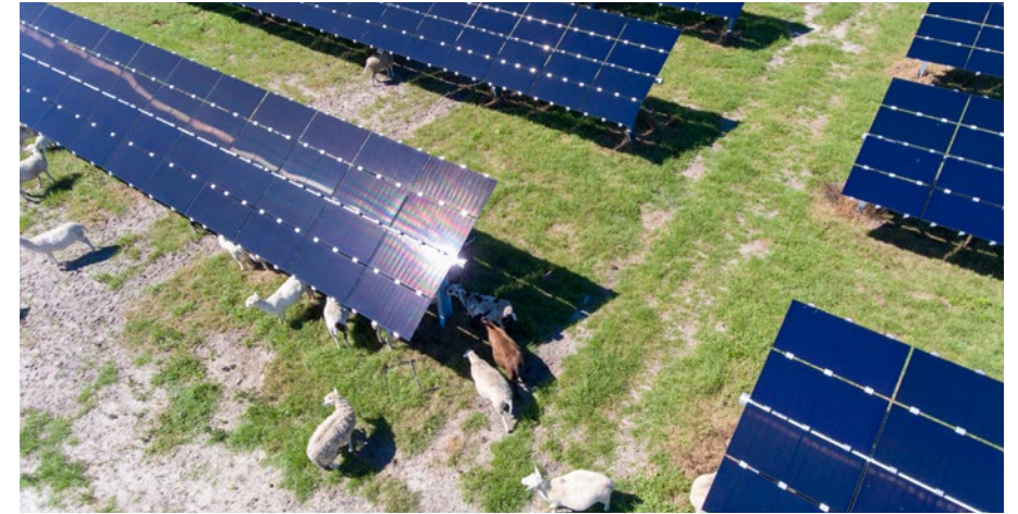
Sheep are an environmentally friendly way to keep the grass short around the more than 740,000 solar panels at Tampa Electric's Lithia Solar facility.
