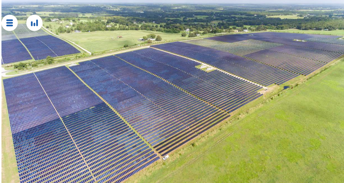
An aerial view of Tampa Electric's Mountain View solar site that went into service in 2023.
